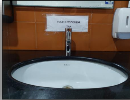
Foot & sensor operated taps for wash basins
