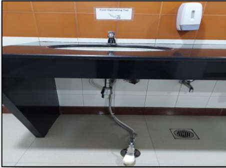
Foot & sensor operated taps for wash basins
