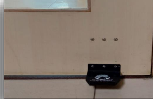
Foot operated door opener/closure
